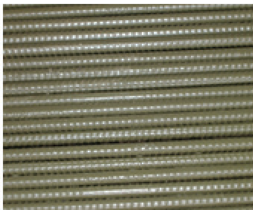
a. CPCC rebars at site
