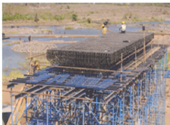
b. CPCC rebars in DFCC Vaitarna to Surat
